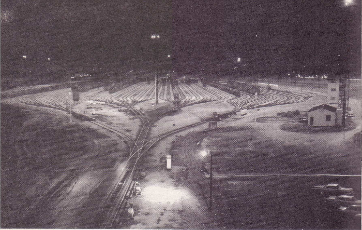
Night view of the Company's new electronic retarder yard at Tulsa, Oklahoma.
