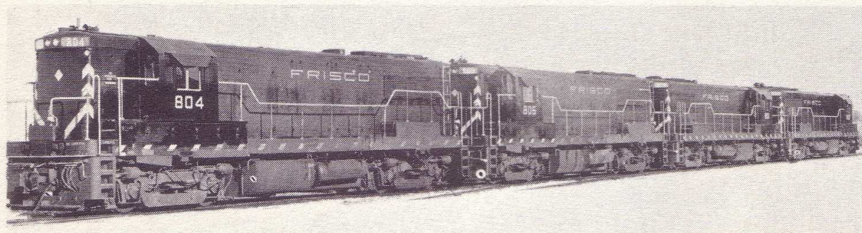
1961 diesel-electric locomotive. Four units together are capable of 10,000 horsepower.
