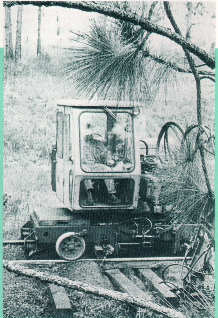
Modern machinery speeds maintenance-of-way work and provides a better roadway.
